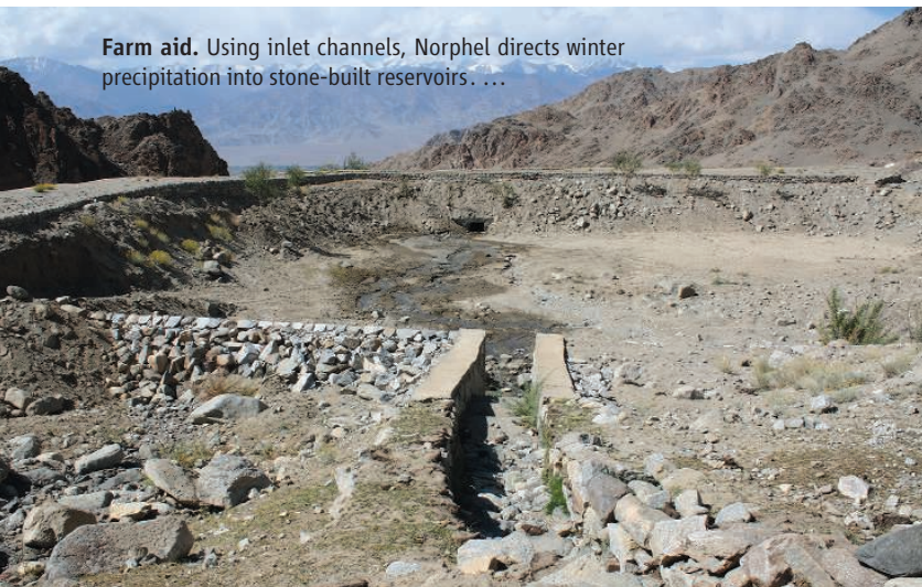
The stored water freezes into an artificial glacier and in the spring, outlets direct meltwater into irrigation. ...
